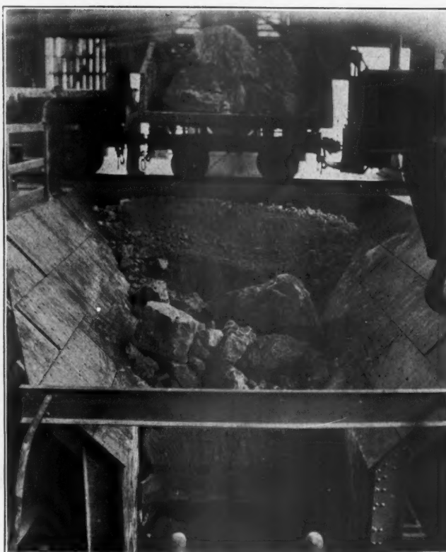
Discharge to Initial Crusher.
